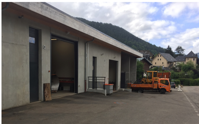
Centre Technique Municipal
